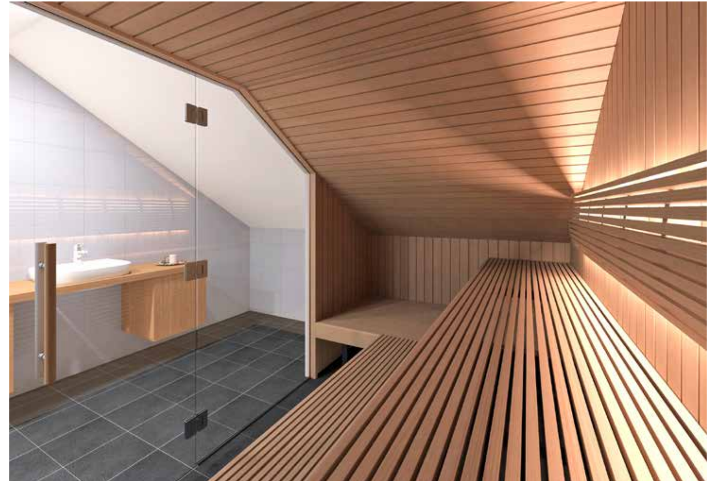
With a little ingenuity, a sauna can fit anywhere; natural alder – walls STS 15 x 90 mm and benches SHP 27 x 27 mm. PRIVATE SAUNA, GERMANY
