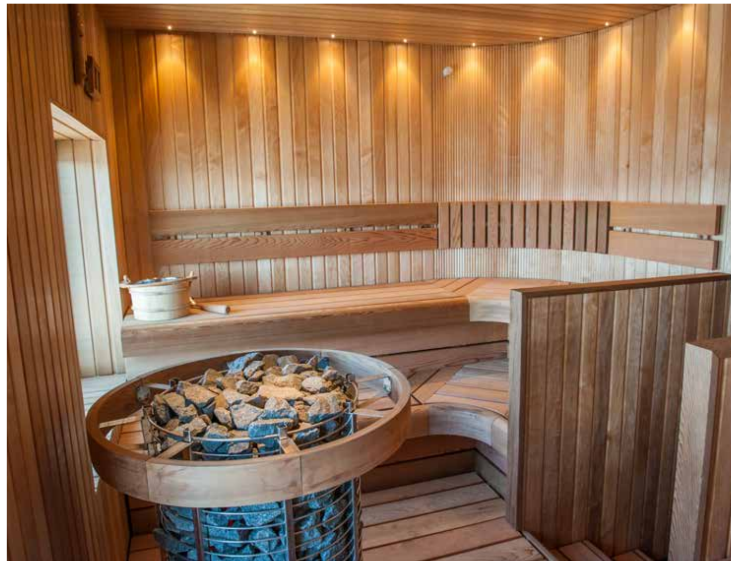
A special design with thermally modified aspen wall panels, STP 15 x 90 mm alongside SRP 15 x 82 mm, and thermally modified radiata pine bench modules SHP 26 x 140 mm. QUALITY HOTEL LAPLAND, SWEDEN
